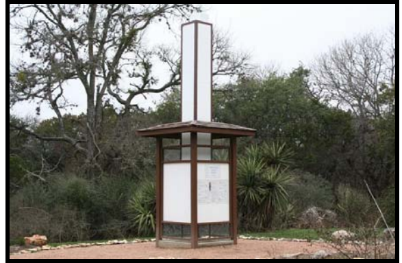
Mayfield Park Tower with smooth siding and metal corners Photo by Kelly Applegate
