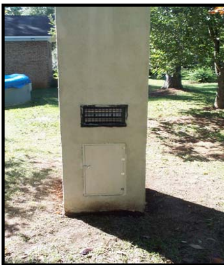
Door and vent detail on coated tower Photo by Dan Howie
